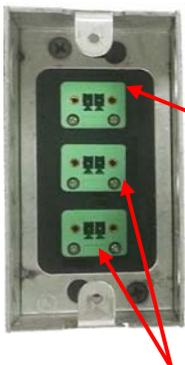
2 position Phoenix connector for audio output to one (1) **Channel 1 (Zone 1)** passive speaker. (Same channel as the active speaker)
